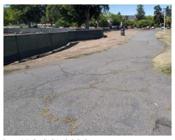
Image 2-7: Cracked Asphalt Path
